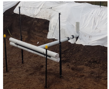
Figure 78: Decanting earth bund system and close up of T-bar dewatering device.
