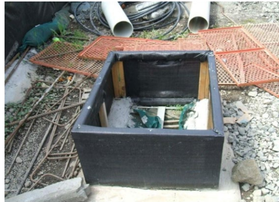
Figure 97: Stormwater inlet protection silt fence within a construction yard
