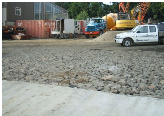
Figure 35: Stabilised entranceway
